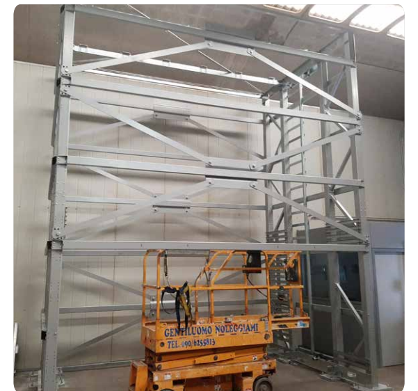
REINFORCED EARTHQUAKE-RESISTANT STRUCTURE
