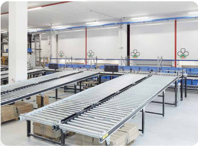
CONVEYOR BELTS AND ROLLER UNITS
